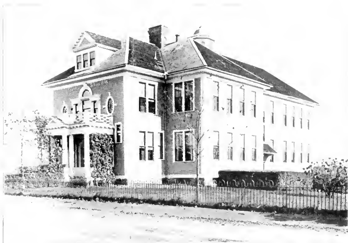
TOWN PLOT SCHOOL. A DISTRICT TYPE OF BUILDING. WATERBURY
